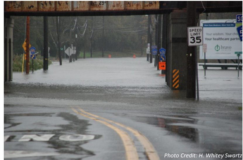
Flooded Roadways in Absecon
