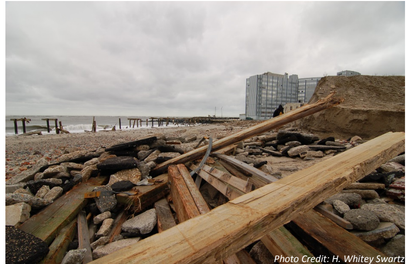
Atlantic City Boardwalk Damage
