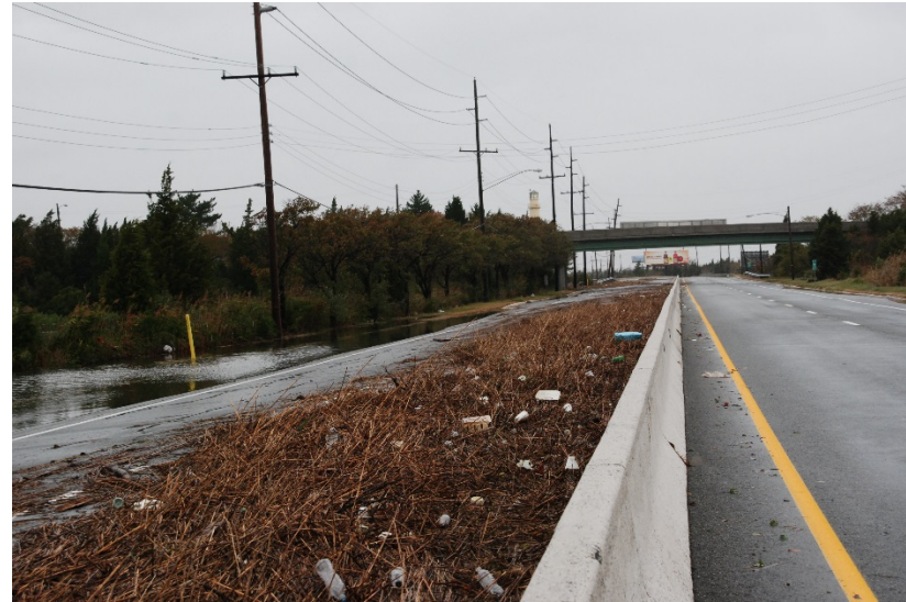
Storm Debris on US Route 40 near Atlantic City
