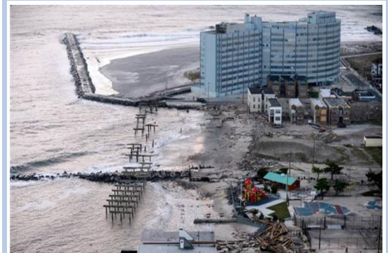
A boardwalk and waterfront property were heavily damaged following Hurricane Sandy in Atlantic City, N.J. One year later, some businesses are still unprepared for disaster, while others have been spurred to make changes. © MICHAEL REYNOLDS
