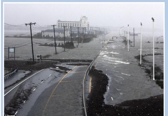
U.S. Route 30, the White Horse Pike, one of three major approaches to Atlantic City, New Jersey, is covered with water from Absecon Bay during the approach of Hurricane Sandy
