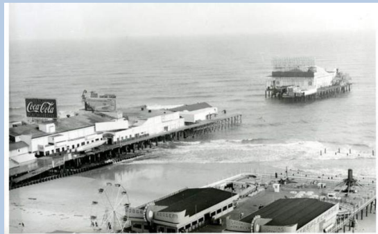
The March 1962 Nor'easter destroyed a section of the Steel Pier in Atlantic City (Photo courtesy of the archives of the Daily Journal).
