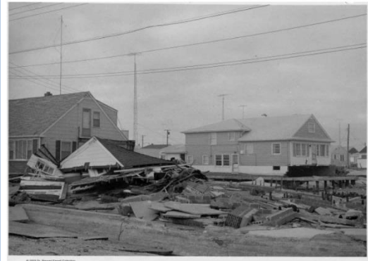
Damage in Longport from the March 1962 Nor'easter. Photo courtesy of the Stewart Farrell Collection.
