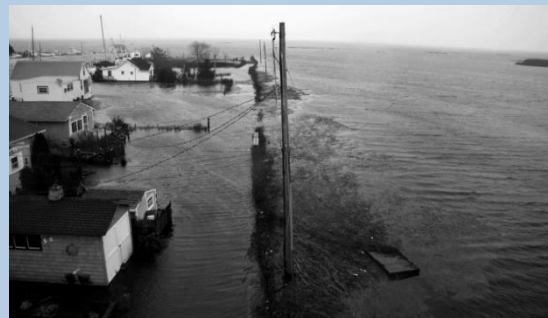
Flooding in Port Republic during a nor'easter on November 13, 2009 (photo courtesy of Flickr user Steve Maciejewski).
