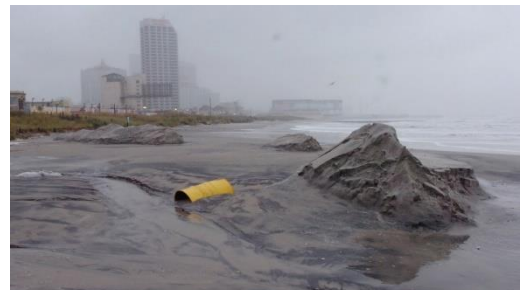
Erosion and damage near Bally's in Atlantic City. Sunday, August 28, 2011. Aftermath of Hurricane Irene. (The Press of Atlantic City/Ben Fogletto)
